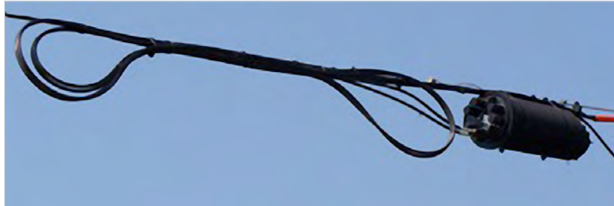
Example: 3-Loop Retrofit Without Storage Devices
